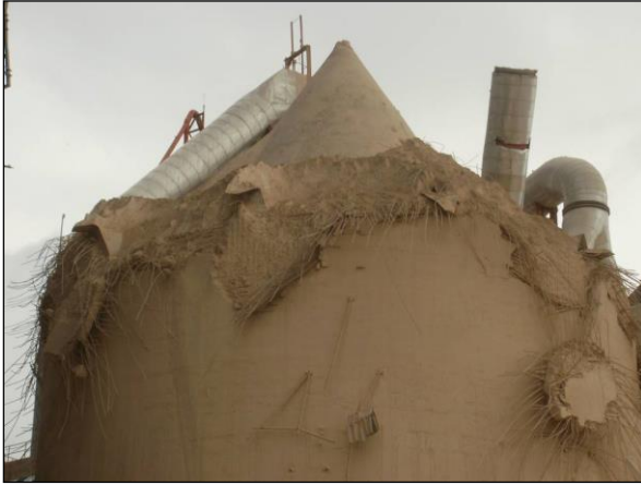
Wall Collapse at about 19.5 to 20.0 m level
