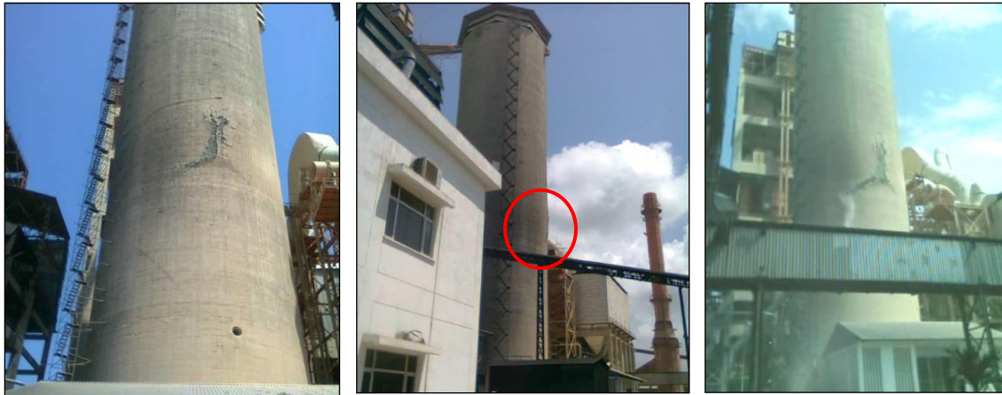
Vertical & Horizontal Crack / split at 30 m to 38 m Level. with a Bulge. Oozing of material Spalling of cover concrete was also observed.
