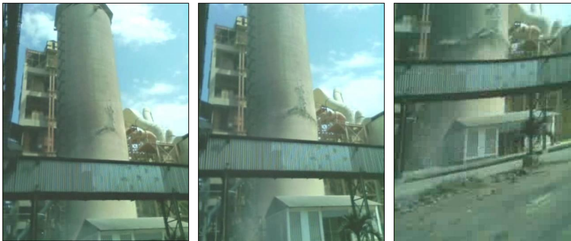
05 Sec before collapse Oozing stopped - 1.00 Sec before collapse Crack widened- 0.25 Sec. On the verge to Collapse
