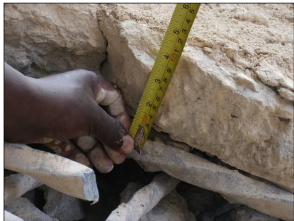
Excessive Cover to the reinforcement at 75 to 100 mm
