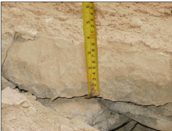
Excessive Cover to the reinforcement at 75 to 100 mm
