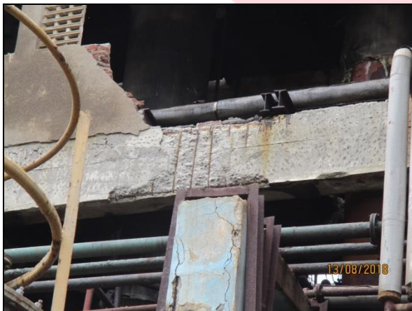
Plaster over RCC member fallen and parapet wall & RCC Grill collapsed due to blast
