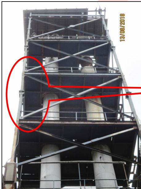
Bend at column joint
