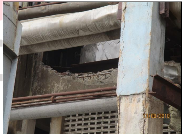
Plaster over RCC member fallen and parapet wall & RCC Grill collapsed due to blast
