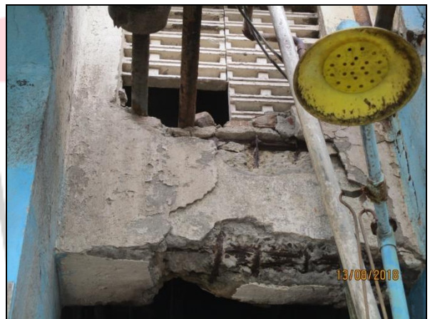
Roof slab adjacent to staircase – crackd and lifted up
