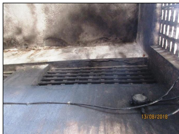
RCC members around blasted area – Ground floor
