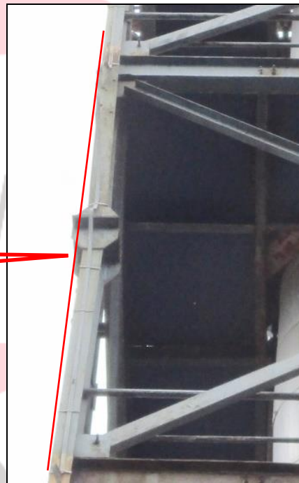
Bend at column joint
