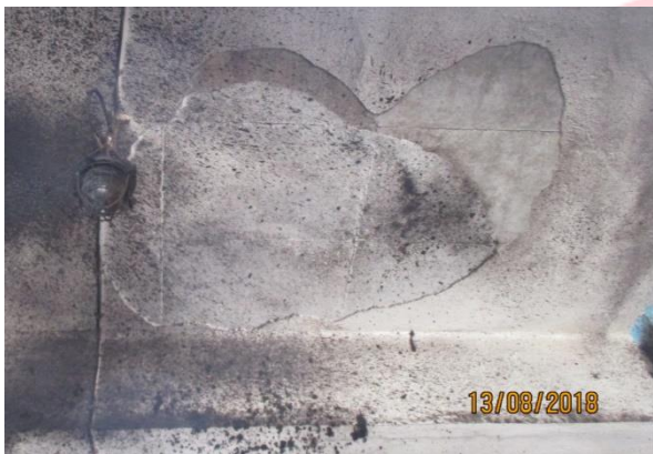
Ceiling plaster fallen due to blast
