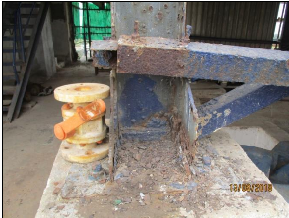
Structural steel members with Severe corrosion
