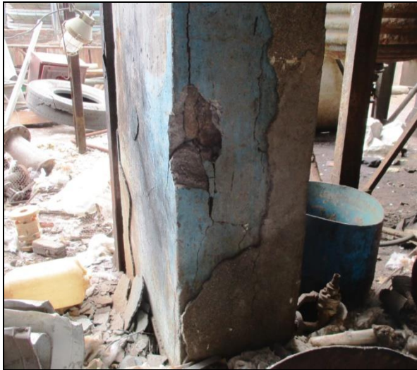
All columns of old building were jacketed with Micro-Concrete 25 to 75 mm thick
