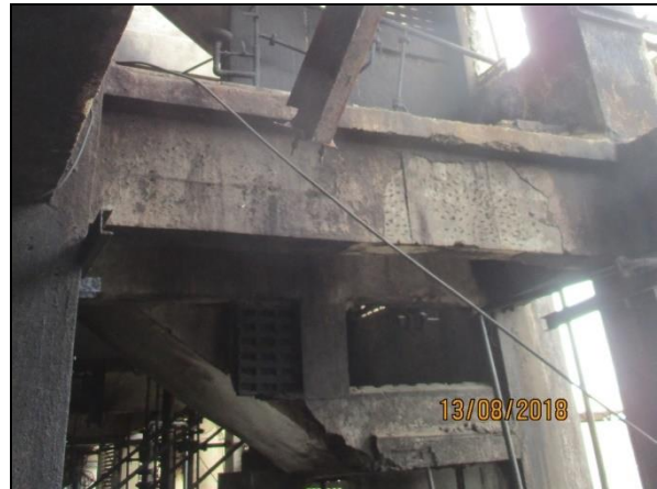
RCC / Steel members around blasted area – First floor
