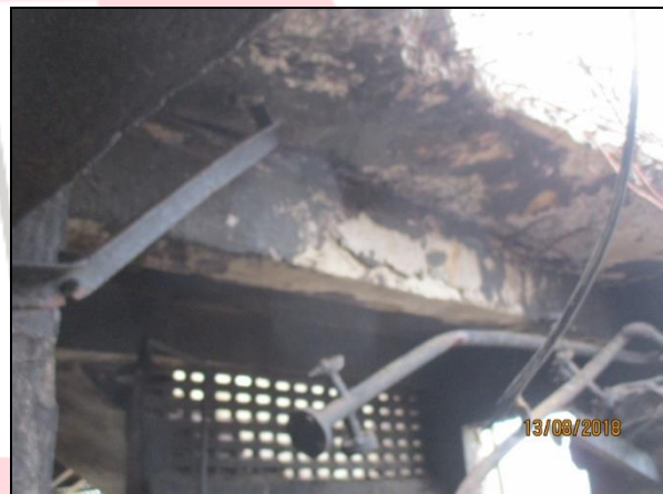
Totally damaged roof slab due to Blast ( Two slab panels )
