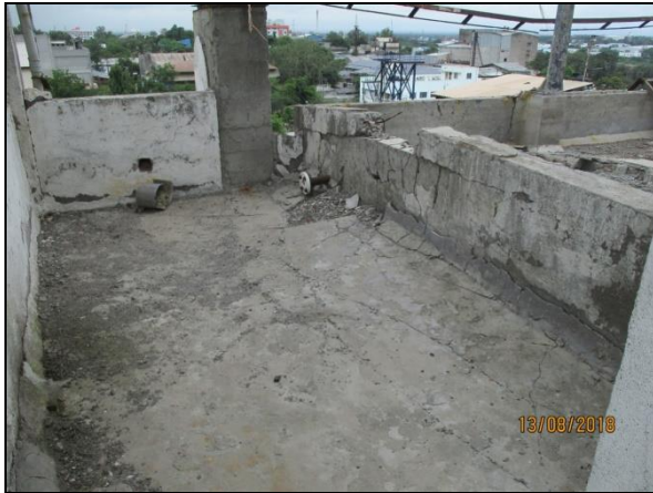
Roof slab adjacent to staircase – crackd and lifted up
