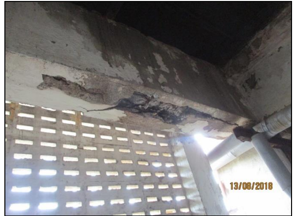
Moderate to Severe corrosion of reinforcement along with spalling of cover concrete
