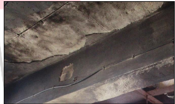
Ceiling plaster fallen due to blast
