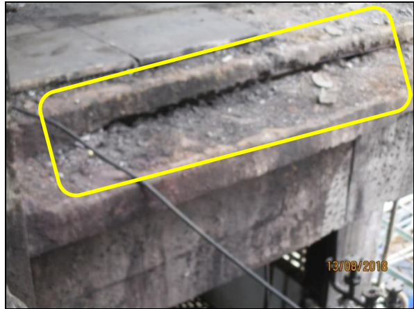
Roof slab adjacent to staircase – crackd and lifted up
