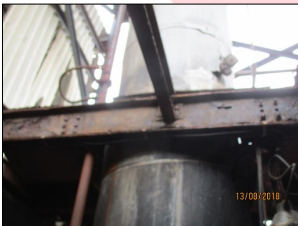
Structural steel members with minor to moderate corrosion
