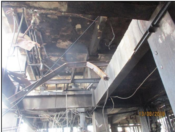
RCC / Steel members around blasted area – First floor
