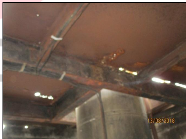
Structural steel members with minor to moderate corrosion
