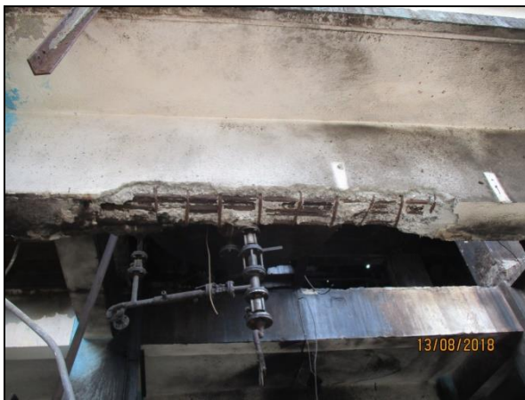
Roof slab adjacent to staircase – crackd and lifted up
