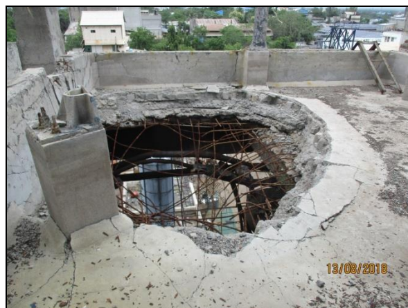
Totally damaged roof slab due to Blast
