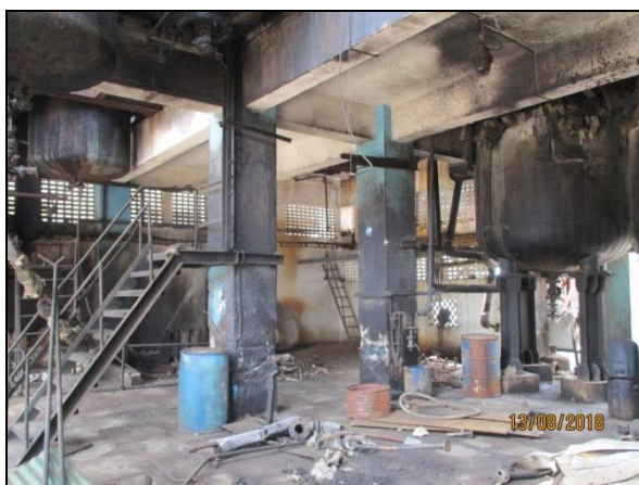
RCC members around blasted area – Ground floor
