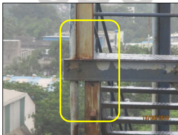
Misaligned Structural Column of staircase of east side Steel tower
