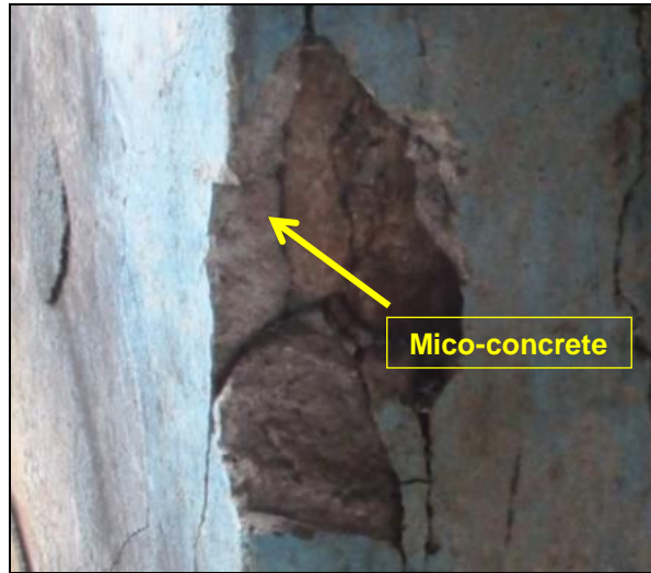
All columns of old building were jacketed with Micro-Concrete 25 to 75 mm thick
