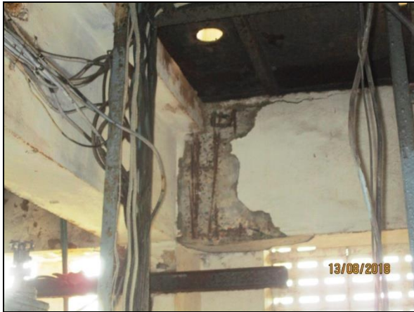
Moderate to Severe corrosion of reinforcement along with spalling of cover concrete
