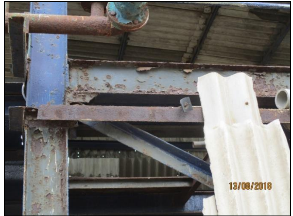
Structural steel members with Severe corrosion
